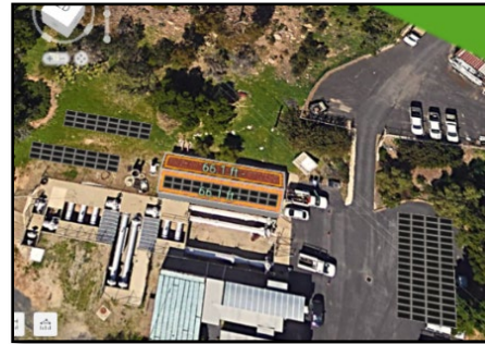
COMB Office Building
