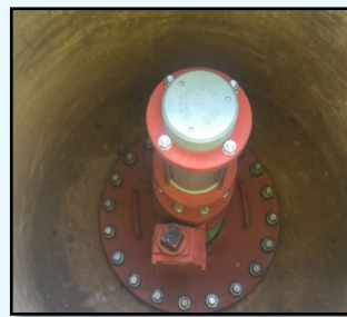
Air Vent 352+07 After
