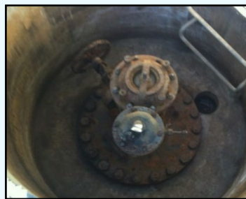
Air Vent 352+07 Before
