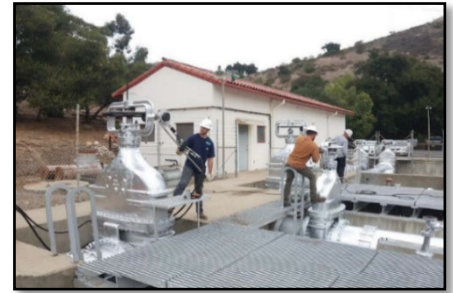
COMB Lauro Control Station
