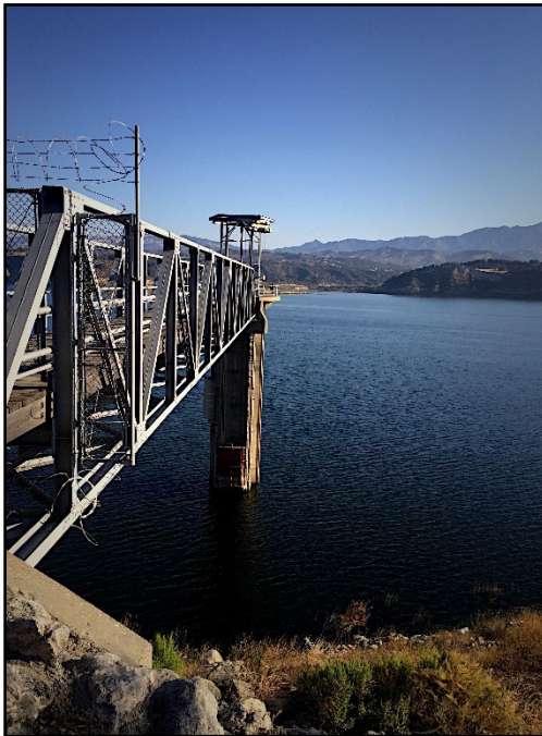
Tecolote Tunnel Intake Tower, Lake Cachuma
