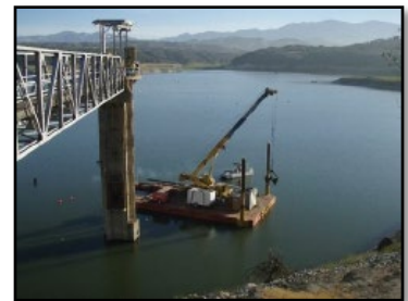
EPF Pumping Facility
