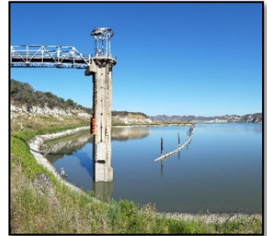
Tecolote Tunnel Intake Tower, Lake Cachuma
