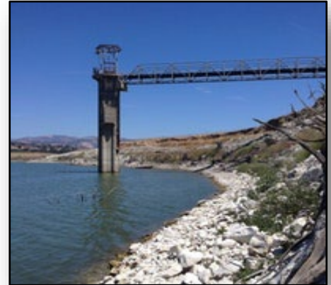
Tecolote Tunnel Intake Tower, Lake Cachuma
